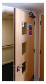
But perhaps the most attractive feature of the LCN 1461, and a key requirement at Birthwaite, is the option for delayed action. This enables the door closing action to be delayed for an adjustable period of time up to a maximum of one minute before resuming normal closing. This allows slow moving traffic to pass through in safety and without disruption.
