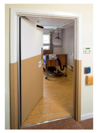
The latest installation is for a resident's room and is operated by a wheelchair mounted proximity sensor or wall mounted push buttons. There is also a key override. The REL 1000 operator is wired to the home's fire alarm system and automatically closes the door after a timed delay in the event of an alarm.
